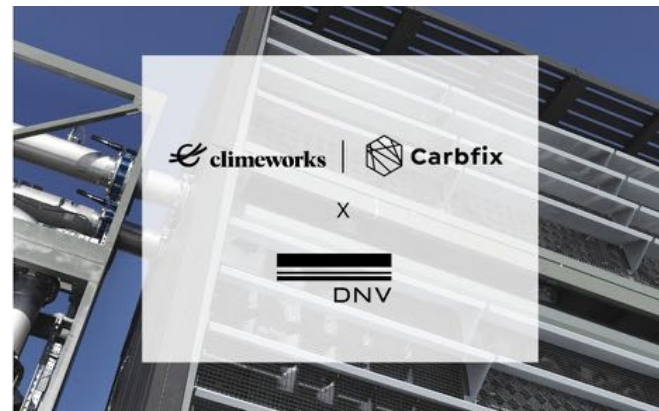
In September 2022, Climeworks and Carbfix announced the development the world's first full-chain certification methodology dedicated to CO 2 removal via direct air capture and underground mineralization storage. This methodology has been validated by DNV. (Image, courtesy Climeworks)
