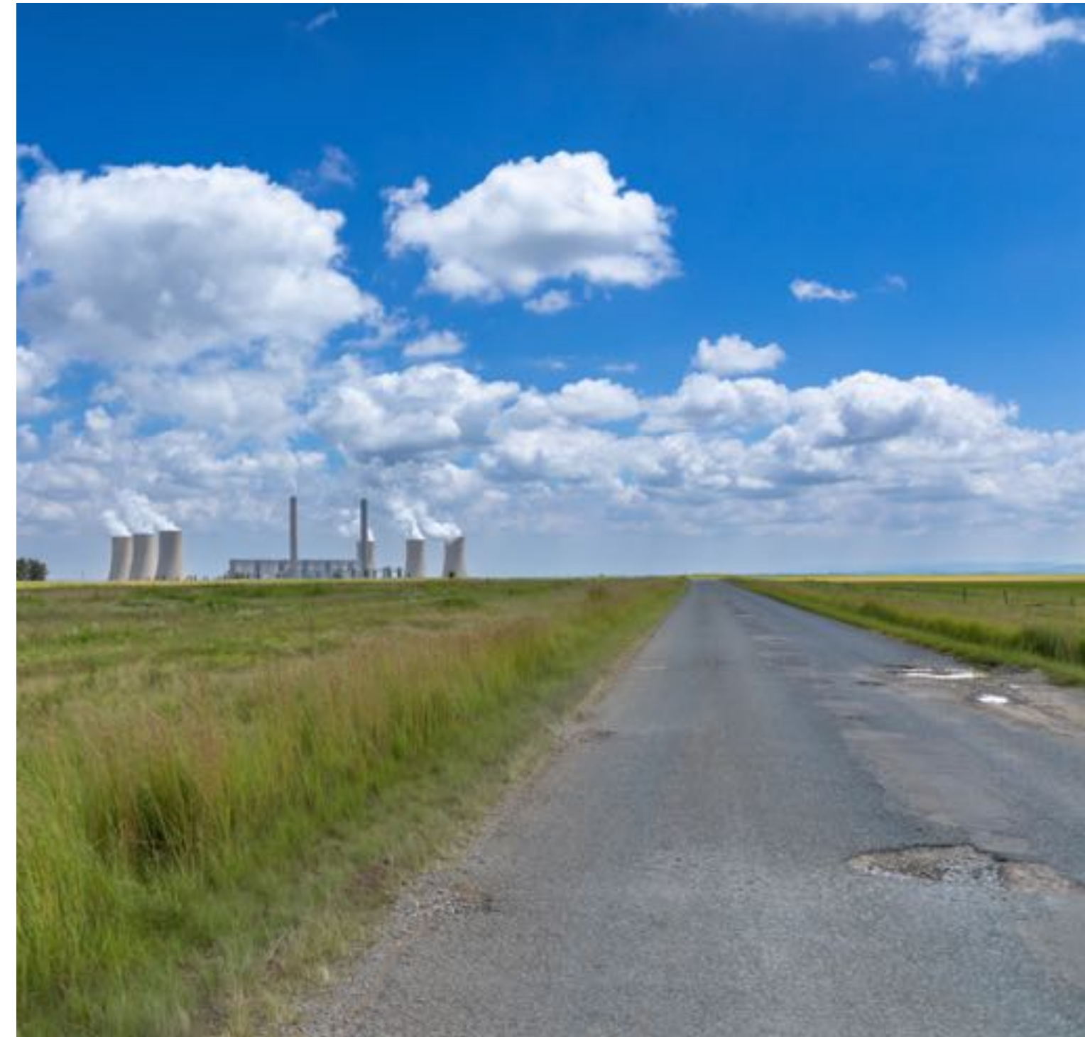
One of 13 coal-fired power plants in South Africa owned and operated by the country's highly indebted utility, Eskom. A rapid, large-scale renewable energy build-out is vital in South Africa to replace the ageing and poorly maintained fleet of coal plants. A lack of generation capacity caused by persistent breakdowns has led to thousands of hours of load shedding in 2022 alone, causing significant hardship and damaging an already-challenged economy.
