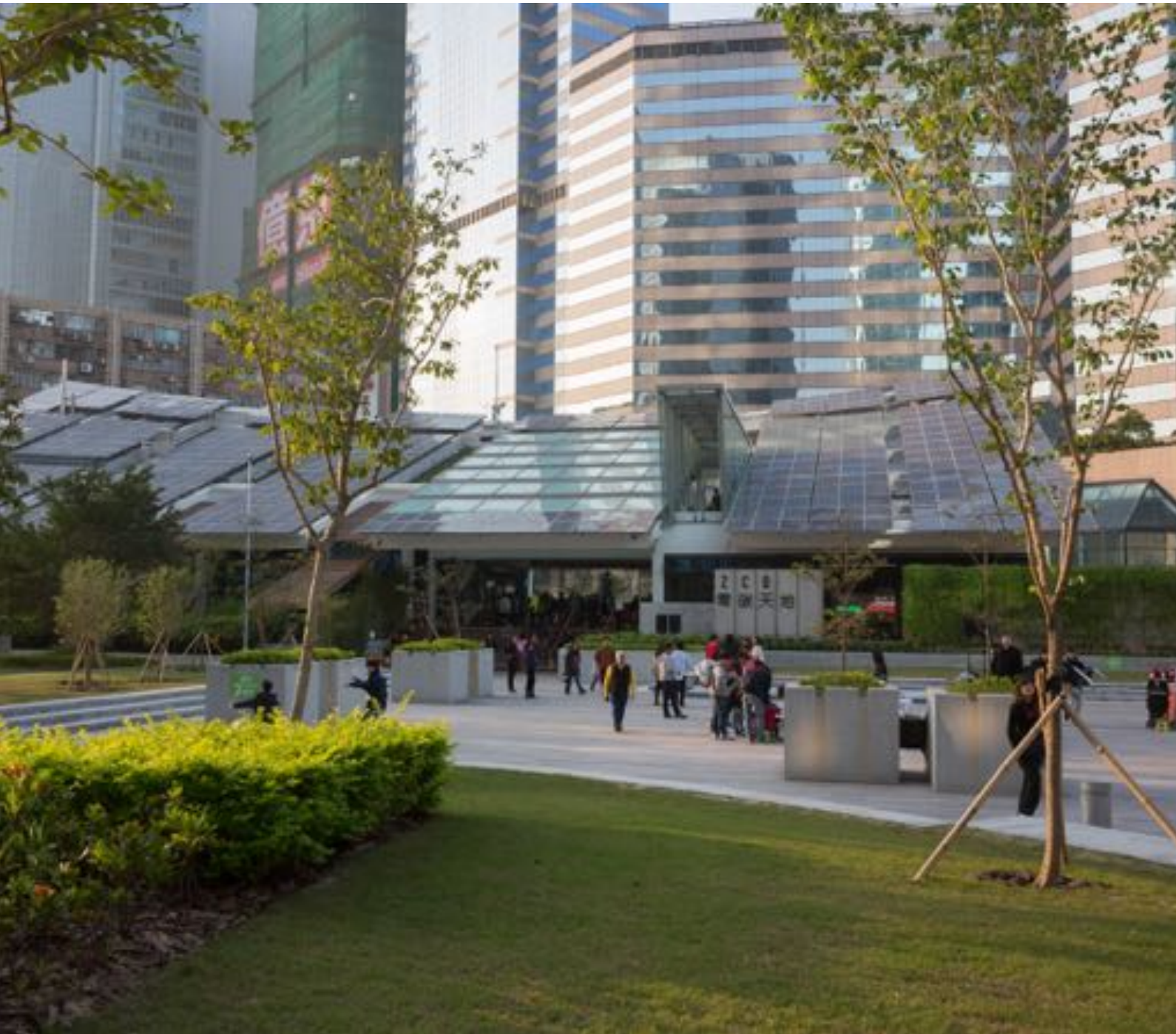
Zero Carbon Building in Hong Kong
