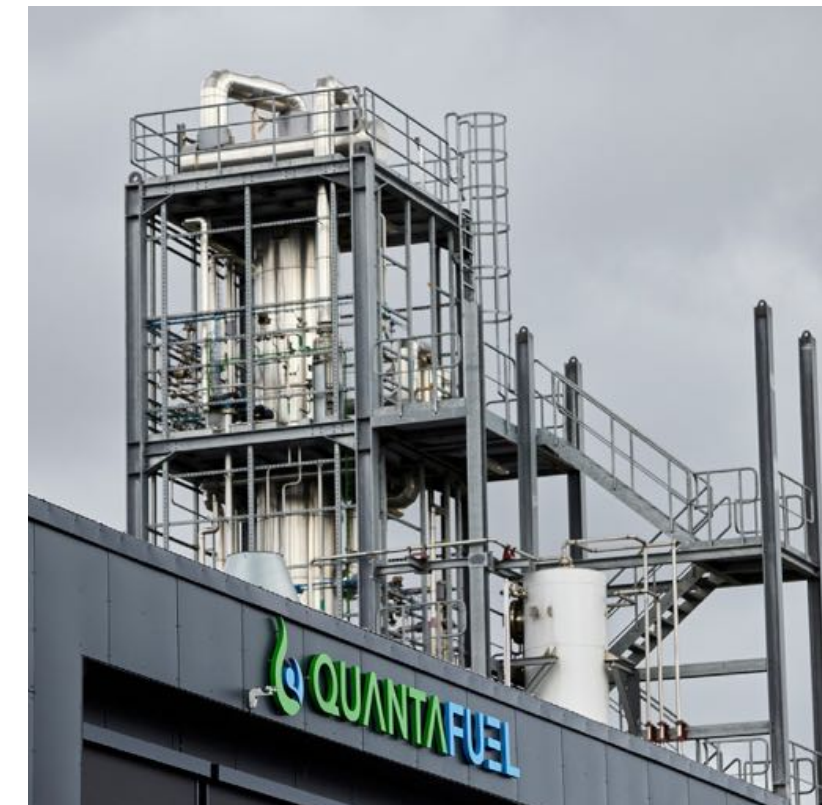
Quantafuel's advanced plastic recycling plant at Skive, Denmark. Image courtesy Quantafuel.
